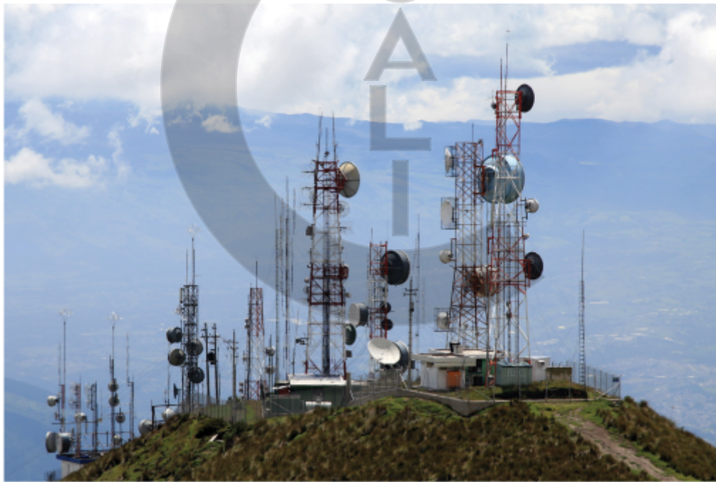
Figure 12.13: These telecommunications masts are situated 4.5 km above sea level in Ecuador. They transmit microwaves, a form of electromagnetic radiation, across the mountain range of the Andes.
