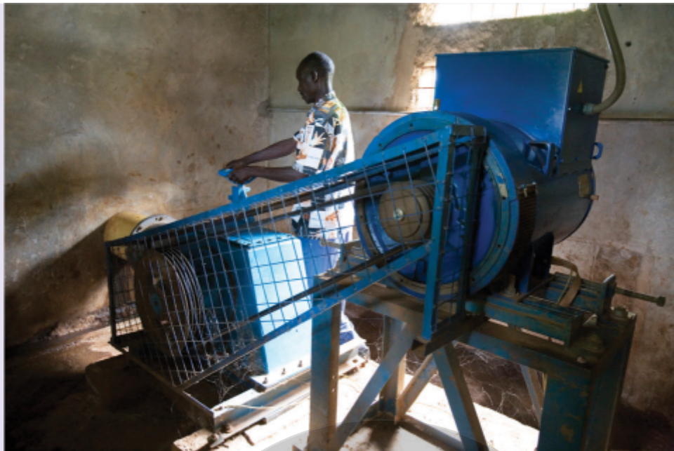
Figure 8.1: An operator controls the water inlet at the Kabiri Falls power plant. The generator is on the right.
