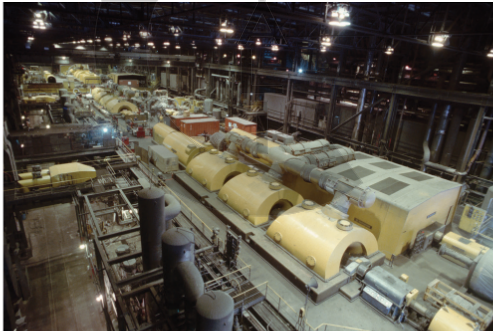
Figure 26.15: For Question 6. The generators of this power station produce electricity at an induced e.m.f. of 25 kV.
