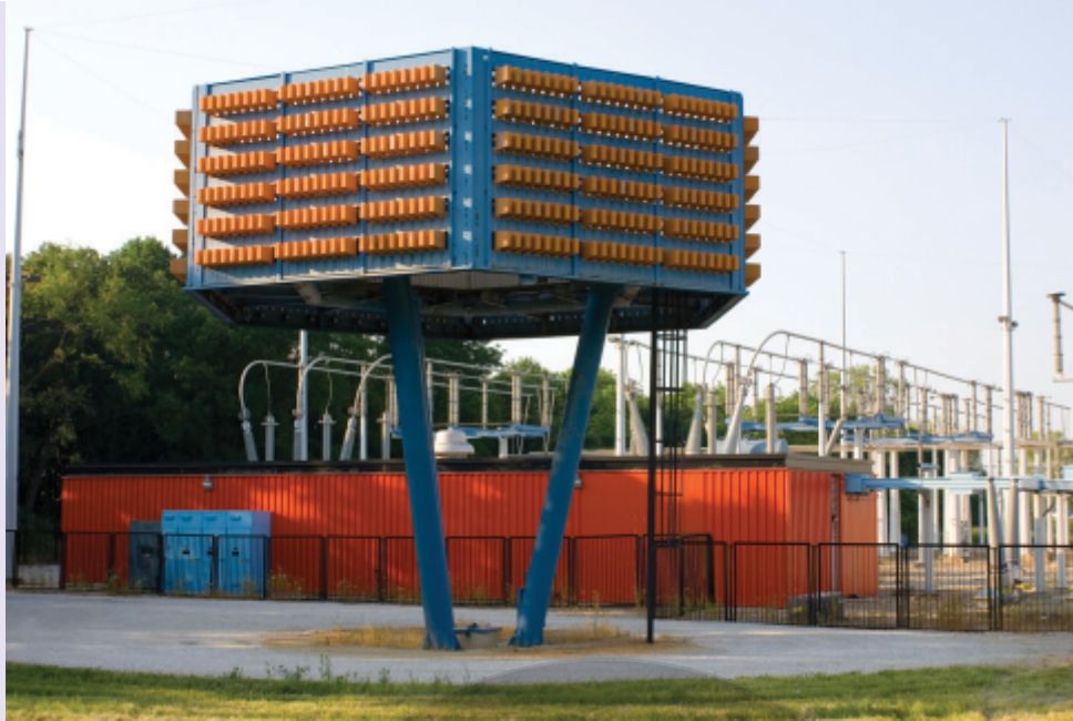
Figure 23.1: One of the world's largest capacitors, built to store energy at the Fermilab particle accelerator.
